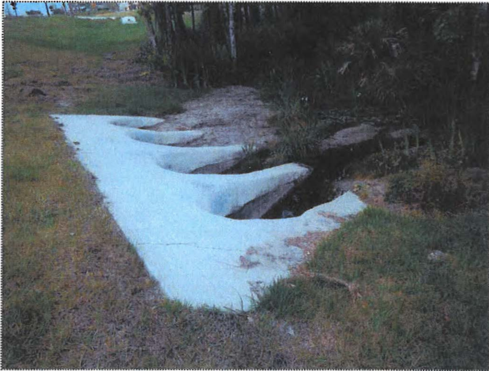
Photo 01. Sand accumulation at north end of quad 36 (April 1, 2019)
